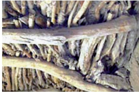
Fig. 13.2. Wood in traditional house (J. N.)
